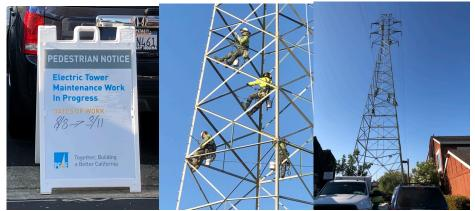
PG&E Crews finished painting the tower on Grenada Lane. This is part of their regular maintenance using non-lead-based paint. Prior to doing the job, they performed an analysis of two soil samples taken from base of the tower. Results: both were under the California residential soil screening level for lead of 80 mg/kg so no soil restoration was recommended.
